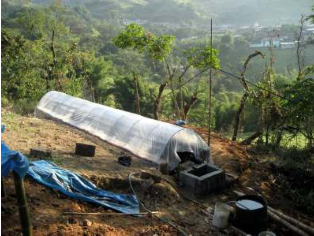
Figure 7: Photo of Taiwanese biodigester installed in Santo Domingo, Piura, Peru (photo from Christopher Galvin).
